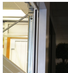
Internal side of steel fixing frame includes a contact ABS strip.
