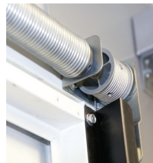
Galvanised torsion spring. Lateral cable pulley.
